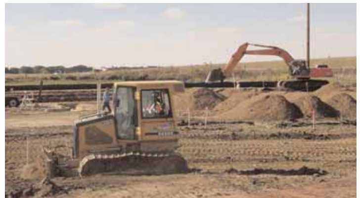
Ground work for the new Hampton Inn, located in Fairmont, MN, began in late September. This will be the third Hampton Inn operated by Torgerson Properties. A grand opening for this 51-unit hotel is scheduled for the spring of 2009.
